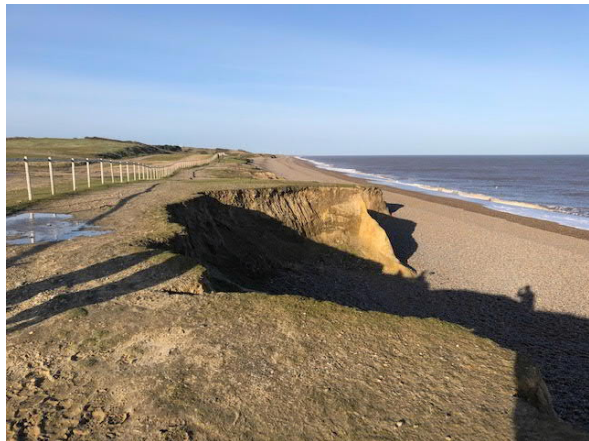
Fig 3.4C. Cliff face condition.
