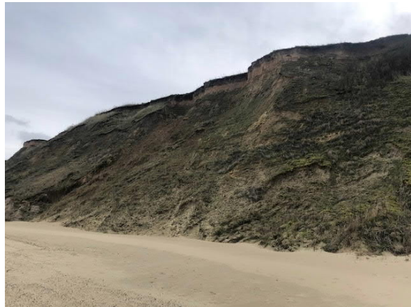
Fig 3.2F. Cliff condition at beach level.
