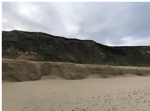
Fig 3.2D. Cliff condition and beach level at HDD.
