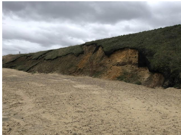
Fig 3.1D. Cliff condition at beach level.
